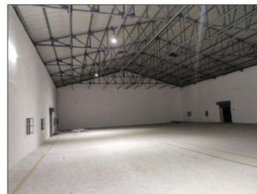
INTERNAL VIEW OF GODOWN
